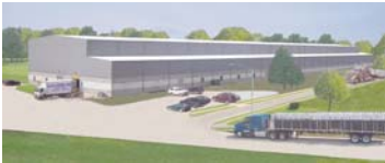
Akron Foundry - Plant 4 1434 Waterloo Rd.
