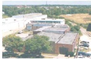
Akron Foundry - Pattern Shop - Plant 2 2705 Wingate Ave.
