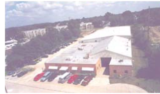
Akron Electric - Plant 3 1025 Eagon St.
